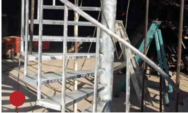
STEEL STAIRS - MINA SALAM
