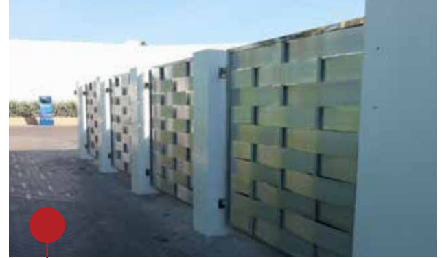
ST STEEL FENCING - JUMEIRAH BEACH
