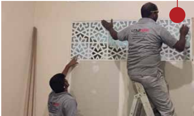
INTERIOR FITOUT - DUBAI INVESTMENT PARK
