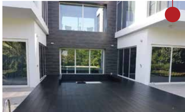
WOODEN DECK - VILLA AL-BARARI
