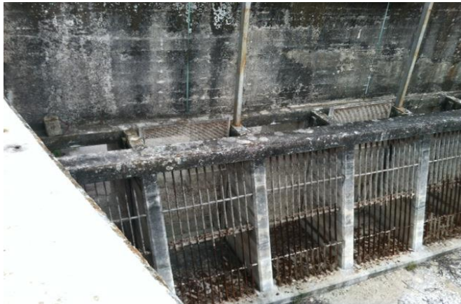
No fish screen on 1, 3, 5 gates. Screen on 2 & 4 gates appear to be inoperable.
