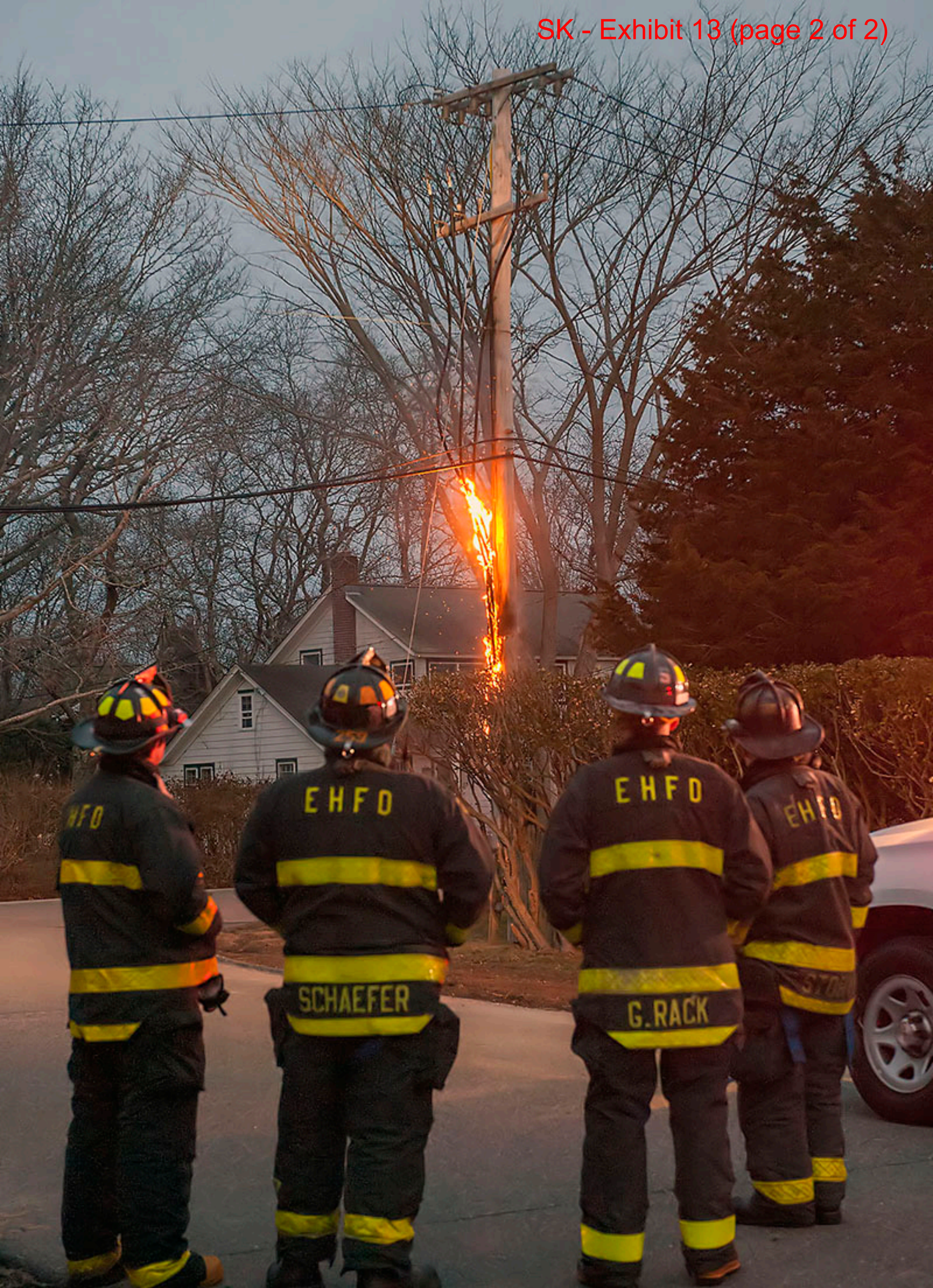
At 5:42 a.m. on Tuesday morning, 2/23/16, the East Hampton Fire Department was dispatched to the corner of Miller Lane and Miller Lane West for a report of a telephone pole on fire. Arriving units were unable to safely attack the fire until PSEG could shut off the power to that system, which they eventually did and the fire was extinguished and the surrounding ground soaked down with a hose line. Photo credit: Michael Heller
