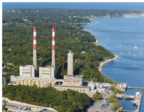
Port Jefferson Power Station
