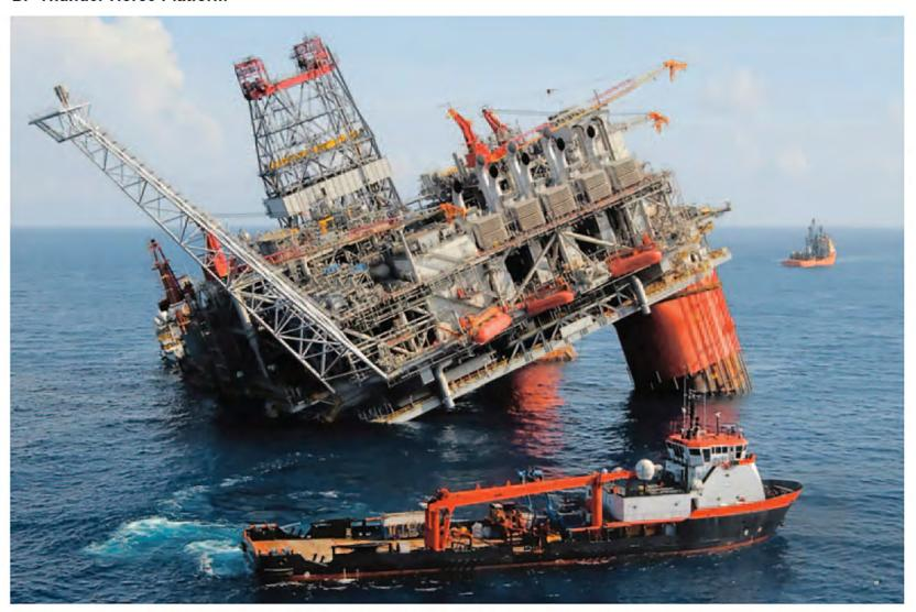
BP's mighty Thunder Horse platform was out-muscled by Hurricane Dennis in 2005 as it was being readied for service. Evacuated crews returned to find the semi-submersible production facility listing badly. After repairs and thorough analysis, additional problems were discovered that put the platform further behind schedule. For BP it was worth the wait: By 2009 Thunder Horse was producing a whopping quarter-million barrels a day.
