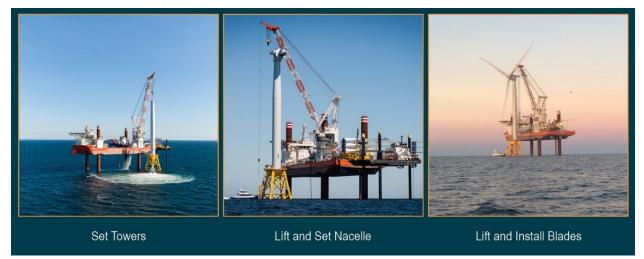
**Figure 3.1-9. South Fork Wind Farm Wind Turbine Generator Installation** *Photographs depicting the wind turbine generator installation sequence.*
