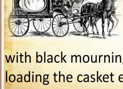
was loaded through a door in the rear of the hearse which was decorated with black mourning draperies. Rollers in the floor made loading the casket easier, and rails and pins kept it in place.
