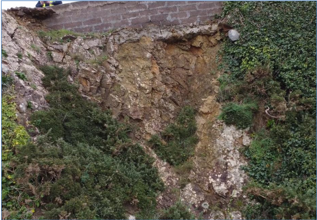
Figure 8 – Close up image of undermined section of La Coupée at Area W3
