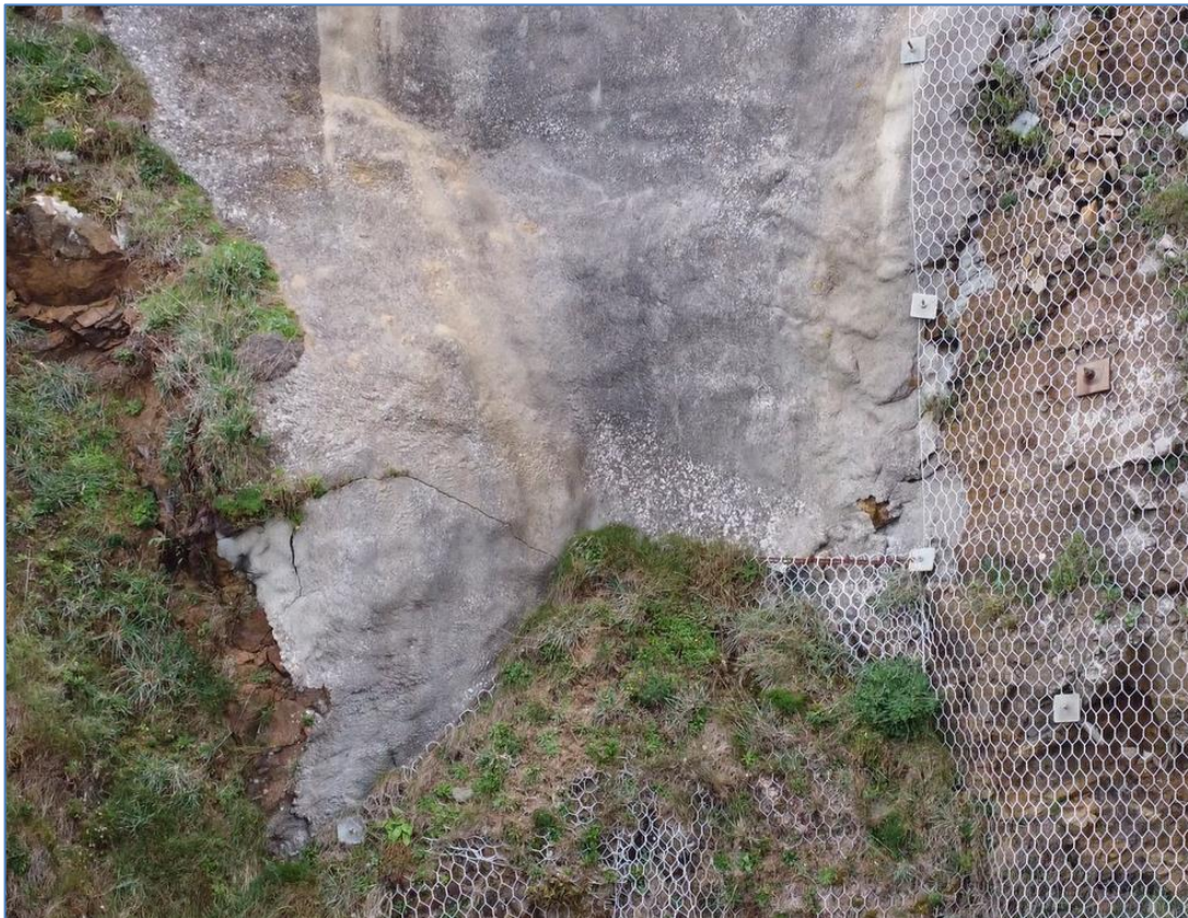
Figure 4 – Close up of cracked shotcrete and several of the corroded element observed on the existing stabilisation
