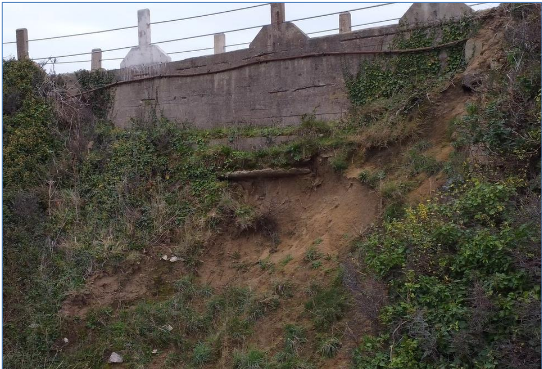
Figure 7 – Close up image of undermined section of La Coupée at Area W2
