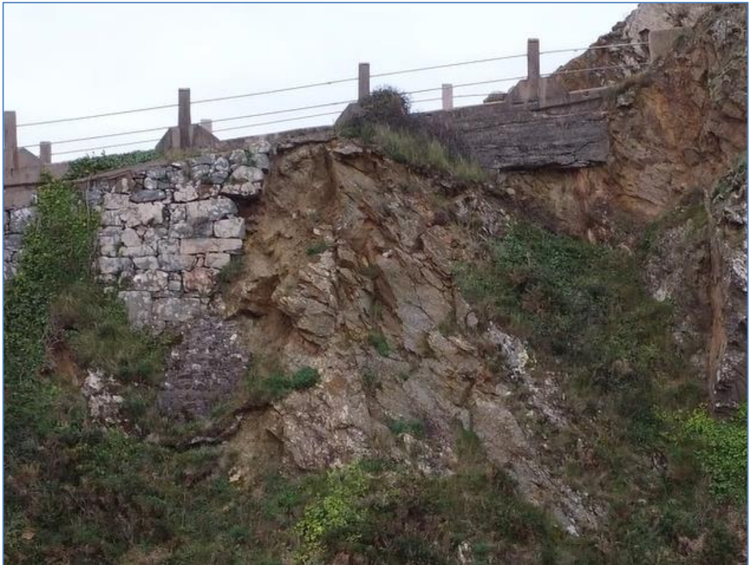
Figure 9 – Close up image of undermined section of La Coupée at Area W5
