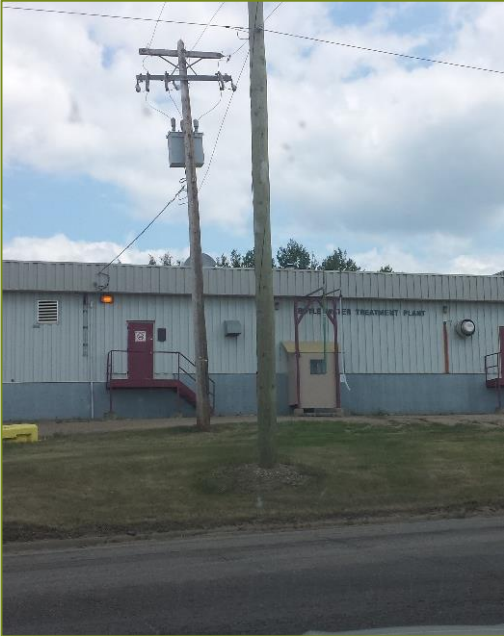
Figure 15. Boyle water treatment plant and fill station
