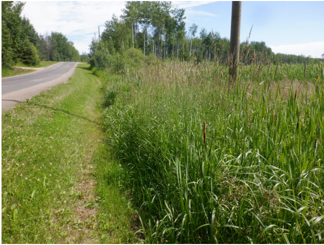
Photo 41: Mowed section on the east side of Bondiss Drive. Standing water present within the ditch.
