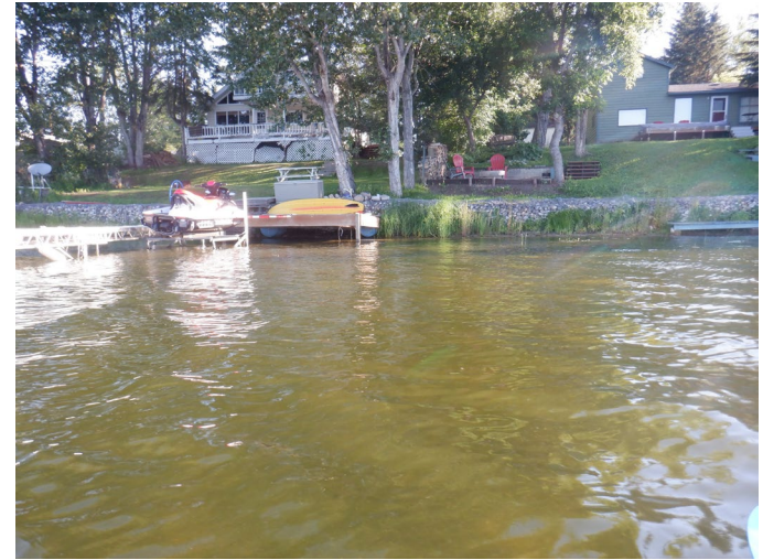
Photo 30: Reach 9 – Retaining wall along shoreline with minimal riparian area.
