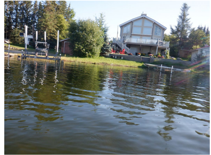
Photo 26: Reach 7 – Lack of emergent vegetation and riparian zone. Typical of high disturbance to shoreline reaches.
