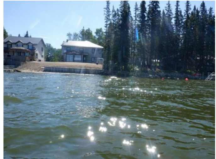
Photo 2: Reach 1 – Retaining wall along developed shoreline. Minimal emergent vegetation. Imported sand along waters edge.
