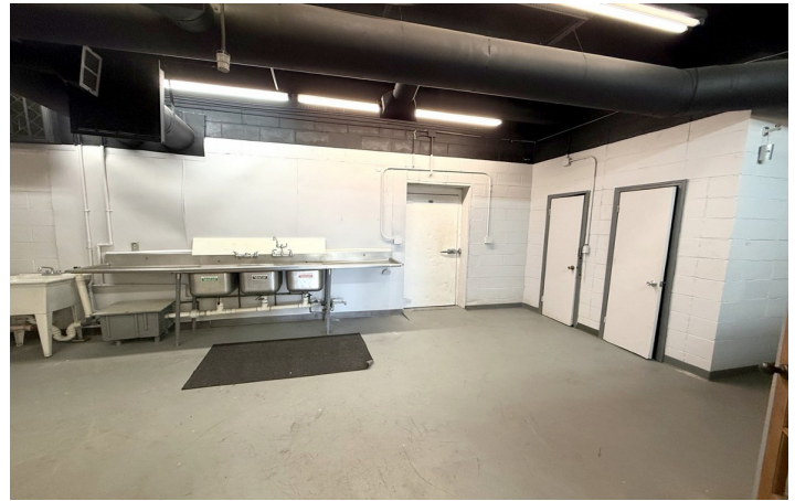
EXISTING SINK / BACK-OF-HOUSE AREA
