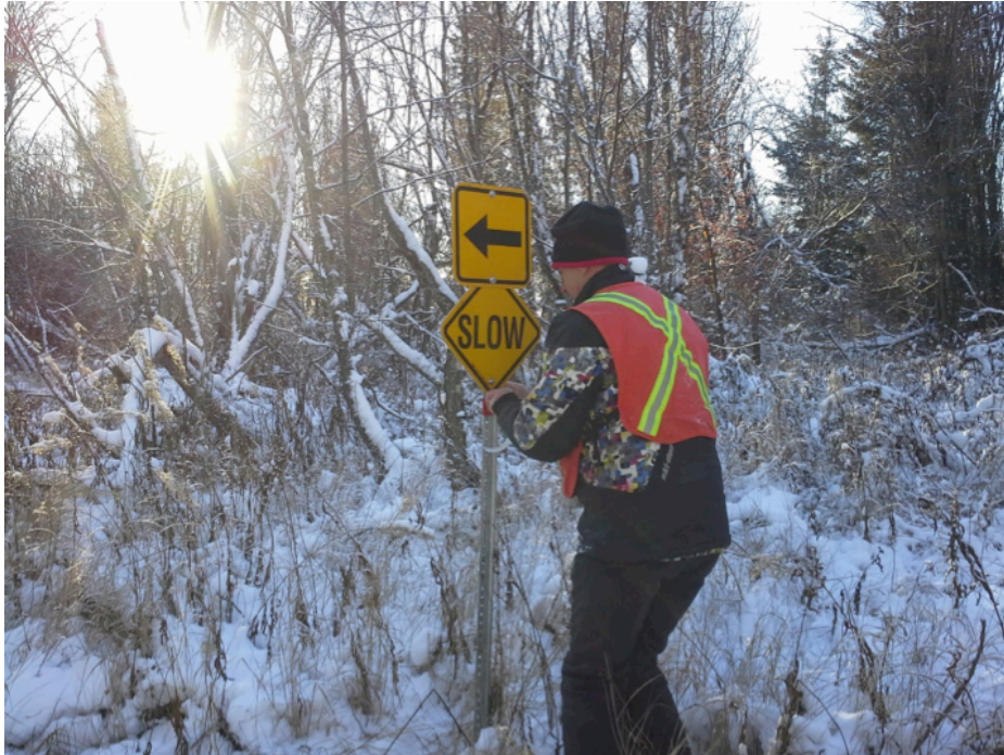
Trail signage installation as part of development, November 2015
