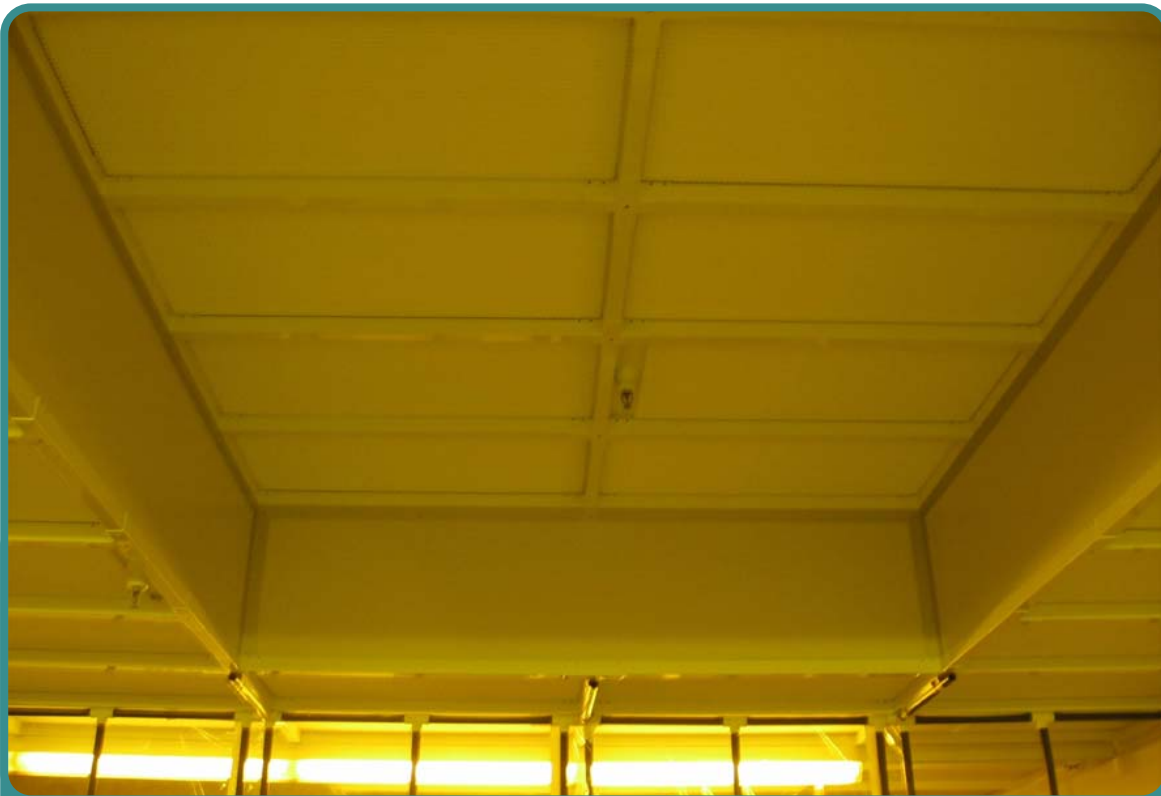
Figure 2. HEPA Filter Installation Complete, Inside Soft Construction Barrier
