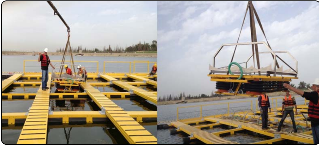
Figure 2 – A Crane Positioning 2 Solar Modules Inside a Platform Cell
