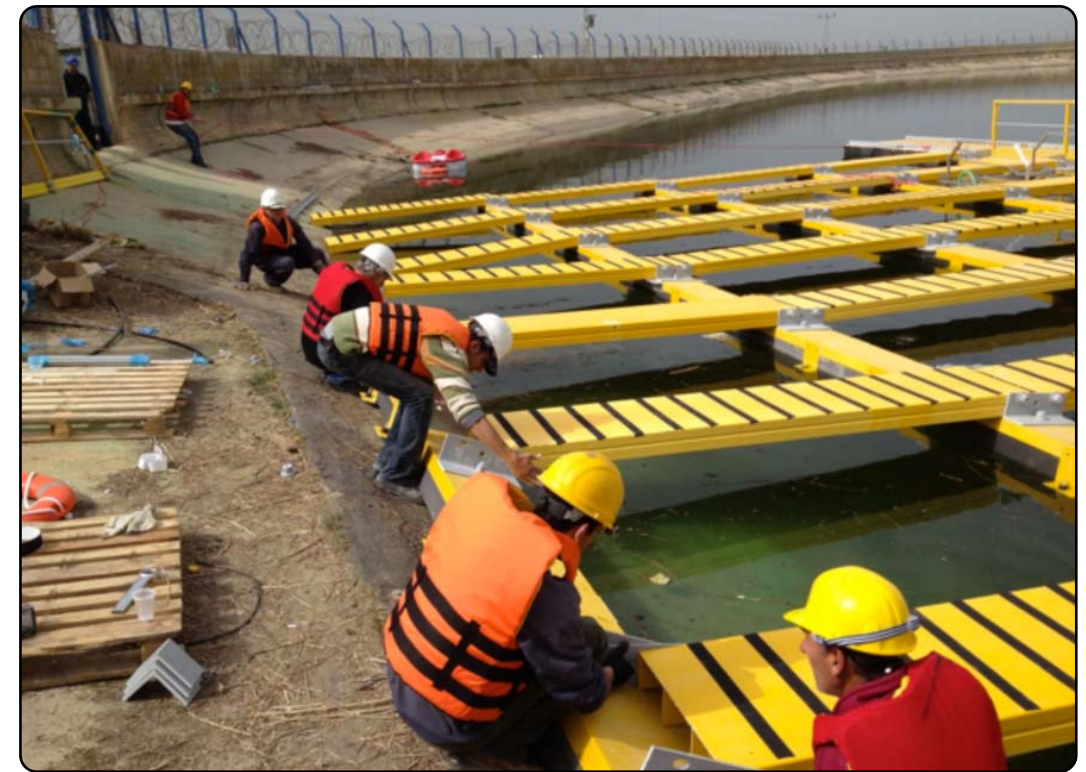
Figure 1 – Assembling the Floating Platform
