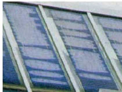
Glass delamination
