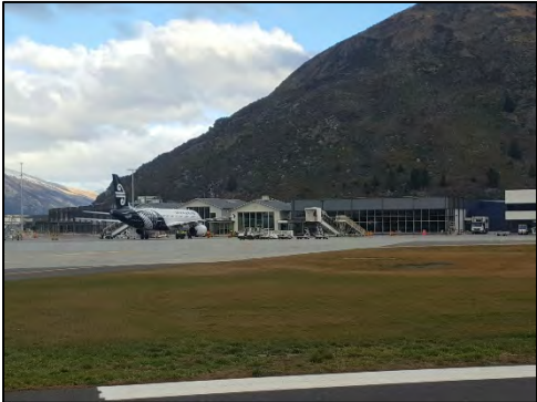
Terminal Building - View from Runway
