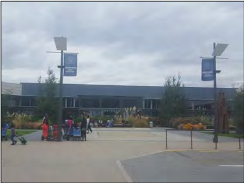
Terminal Building - View from Carpark
