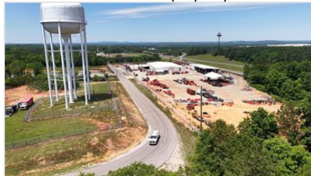
Paved road access
