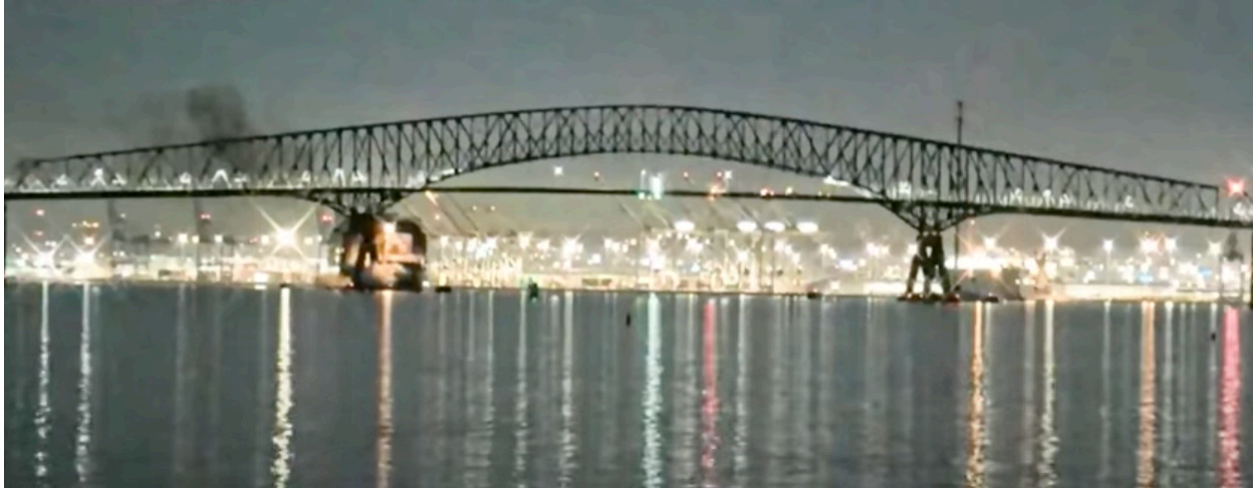
Fig. 7. The Dali crashes into the western pier of the bridge raising a big splash of water between the pier and the ship's bow. The ship's lights appear to turn back on. (StreamTeam Live)
