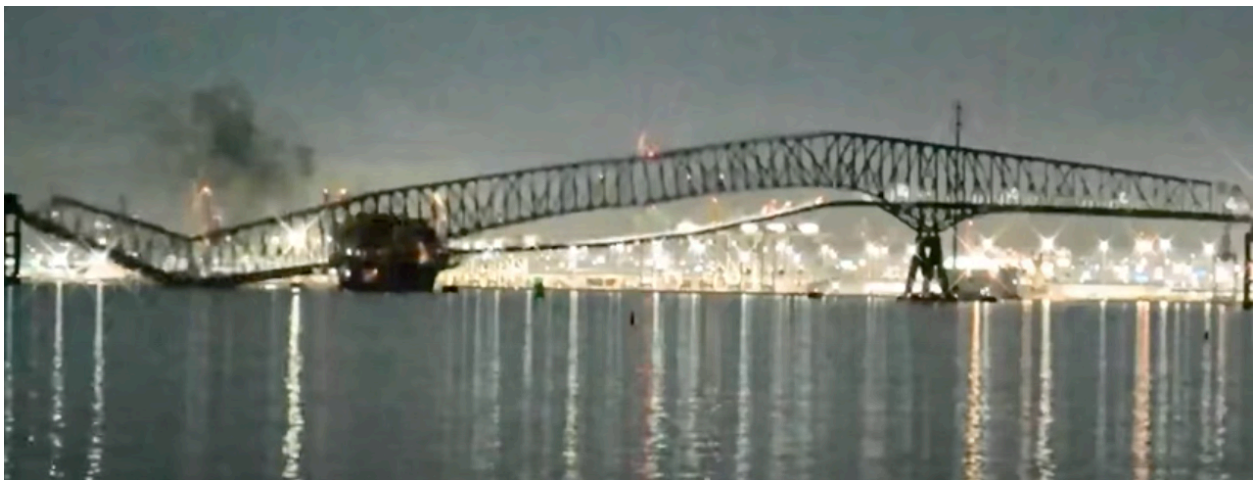
Fig. 8. The bridge begins to collapse after the western pier looks appearing to collapse removing its support of the bridge. (StreamTeam Live)
