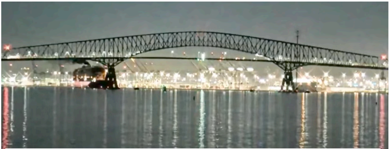
Fig. 5. The container ship, Dali , is approaching the west pier of the Francis Scott Key bridge on the left with all lights appearing to be working alright (StreamTeam Live)
