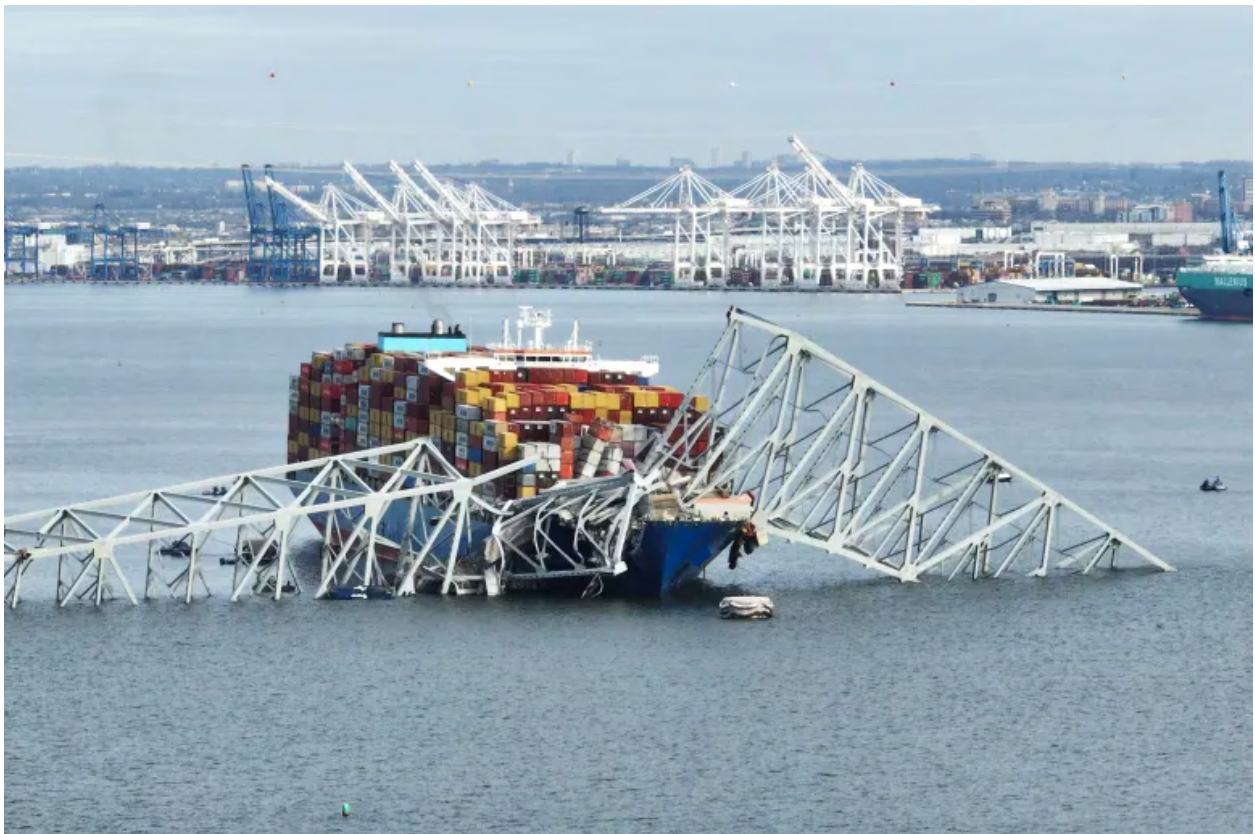
Fig. 10. Daylight aerial view of the remnants of the Francis Scott Key bridge resting on the Dali 's bows'l. (Jim Watson/AFP via Getty Images)
