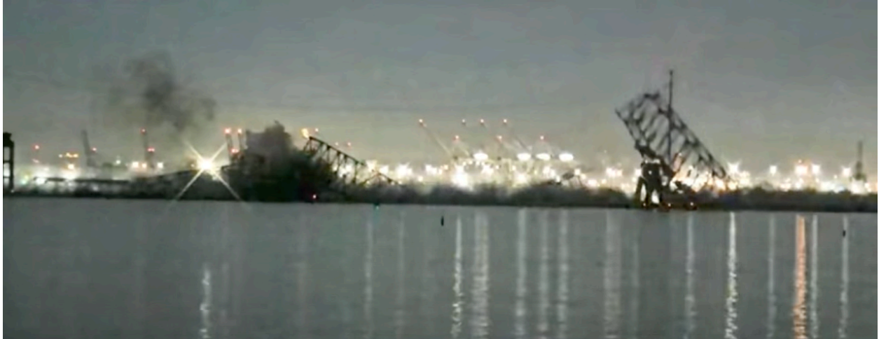
Fig. 9. The bridge completely collapses into the Patapsco River and onto the bow of the Dali . (StreamTeam Live)
