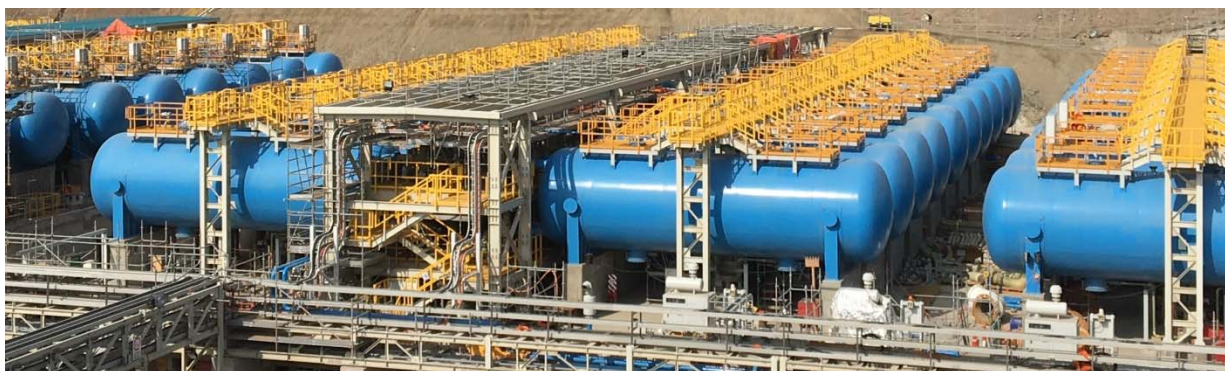
Figure 4: Dual media pressure filters (3D Model and installed filters)
