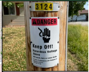
Typical Wooden Pole Location Number. Aluminum and Fiberglass Poles may not have a Location Number on them.
