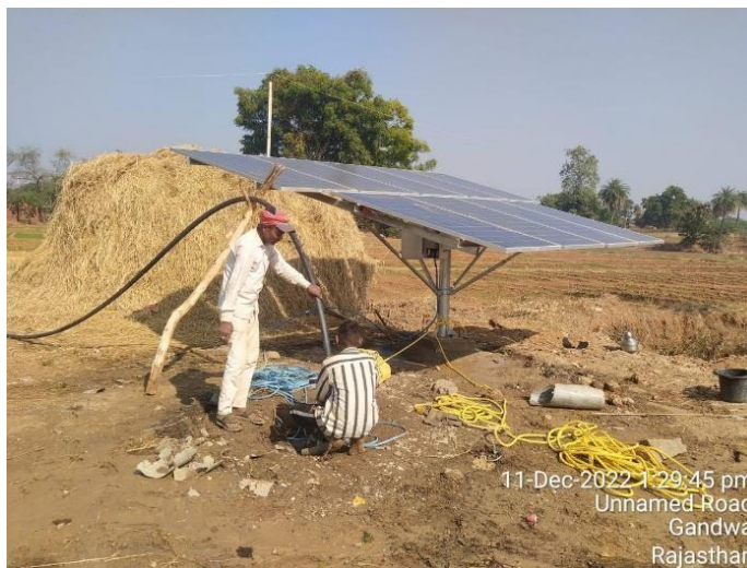
Installation of Panels & Motor
