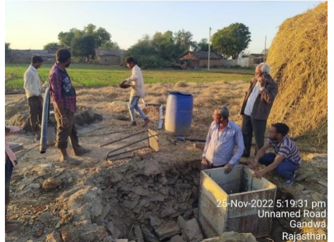
Reinforcement & setting up of Foundation
