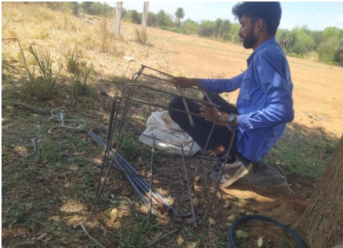
Finalising the Location & Excavation for the Foundation
