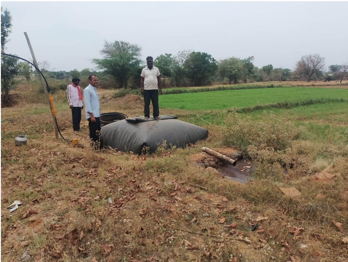
Installation of Bio-Gas Units
