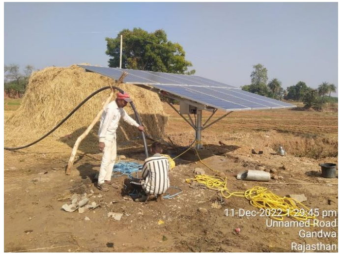
Installation of Panels & Motor
