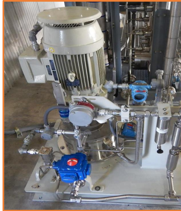
Electric Seal Gas Booster to Avoid Venting (Pressurized Hold)
