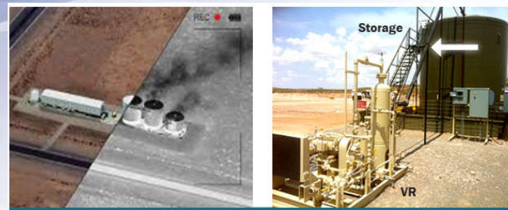
FIGURE 6. Aerial infrared photo showing crude oil tank vent emissions (left) and photo of vapor recovery (VR) unit installed on storage tank to prevent emissions (right, with connection line identified). Photo courtesy of HY-BON/EDI (Source)?
