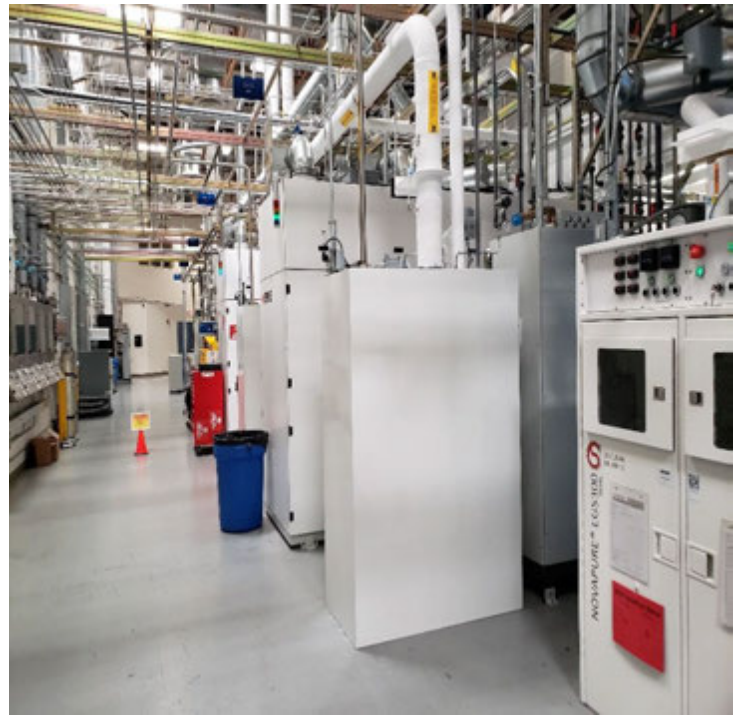
Large Amounts of In-Use Gas Cabinets with Process Piping.
