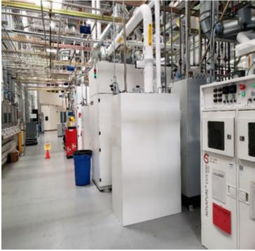
Large Amounts of In-Use Gas Cabinets with Process Piping.
