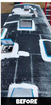
STEP 3: INSTALL THE CRAZY SEAL SYSTEM
