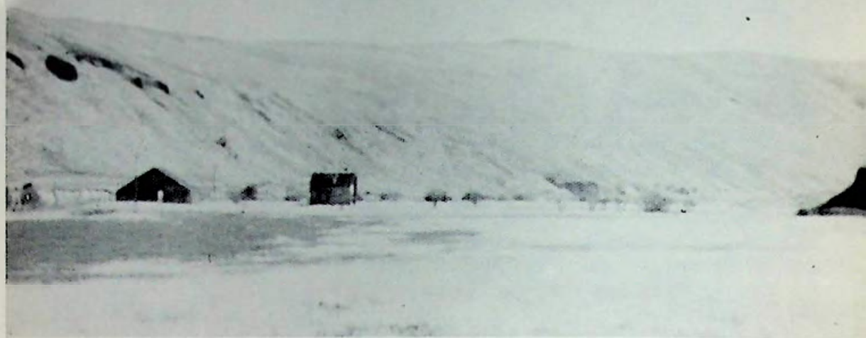
D, above, Frank Chapman shed (now owned by French).
