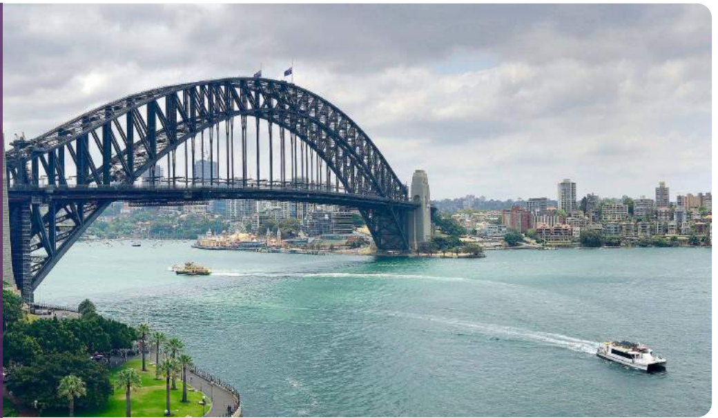
Sydney Harbour Bridge, New South Wales
