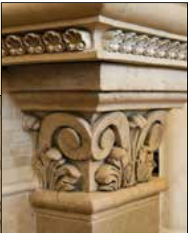
Above and Below: Details of a Neptune fireplace composed of coral stone, cut on-site with Ellison's custom floral panels, capitals, the Neptune insert, and shell borders. Inset: Detail of column support for a bar repeats the shell border motif.
