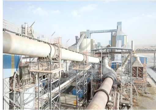
(Photo: ABB Cement)
