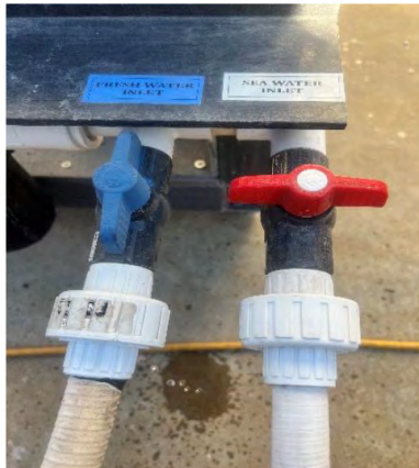
5.1.1.2 Fresh Water Valve On and Sea Water Valve Off
