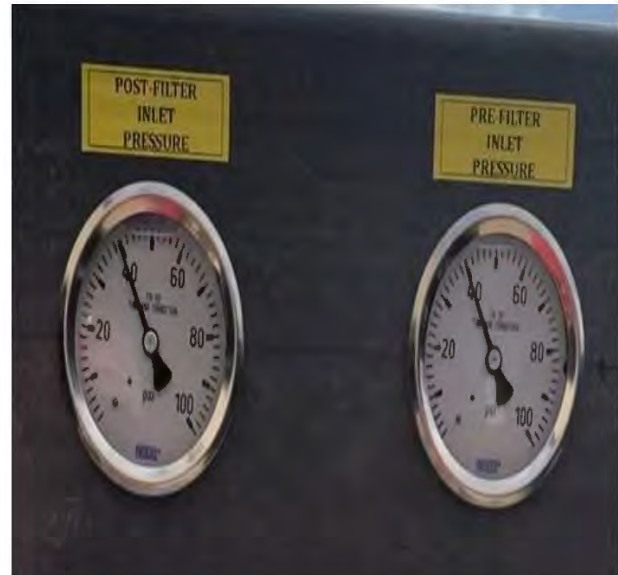
9.2.1.1 20 and 5 Micron Filters and Inlet Pressure Gauges
