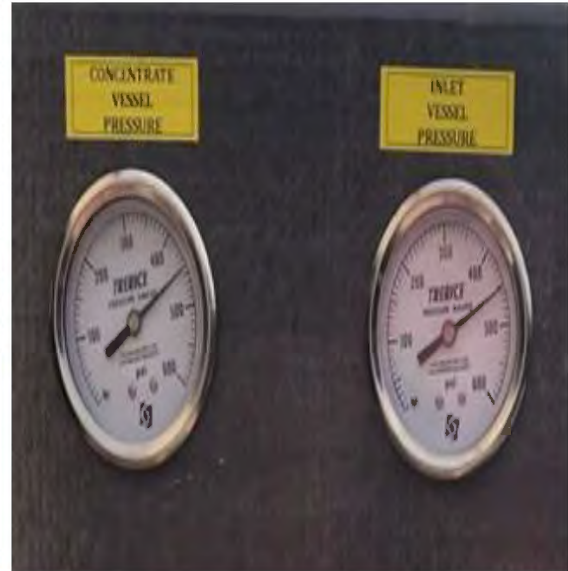
9.3.1.1 RO Membrane and Vessel Pressure Gauges
