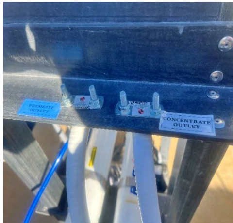
2.4.1.1 Permeate and Concentrate Output Connection Photo
