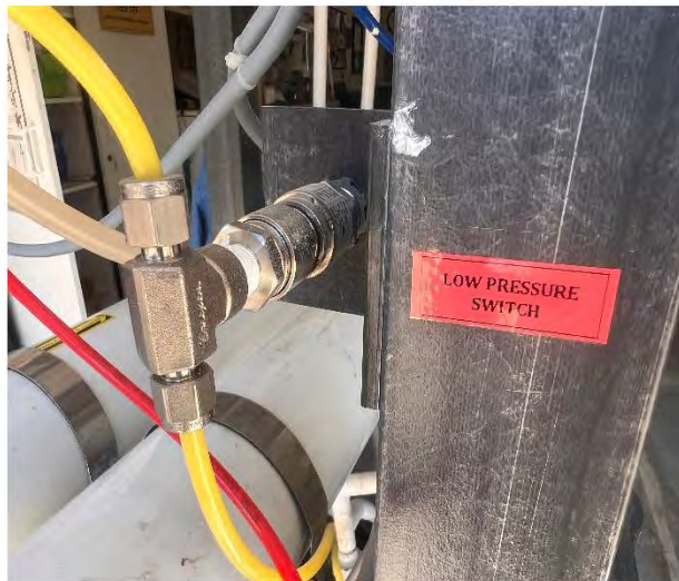
6.2.1.1 High Pressure Pump Inlet Low Pressure Sensor
