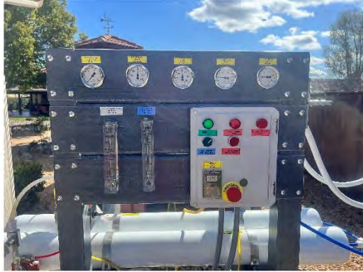
5.2.1.1 Flush Complete Gauge Readings
