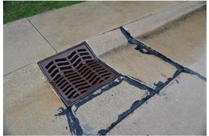
6. View of a storm drain inlet, concrete curb, and common walk along the onsite roadway. Note the black sealant in the roadway joints.
