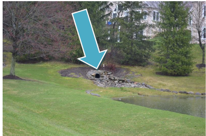
24. View of a storm drain discharge at the pond shown in the previous photo.
