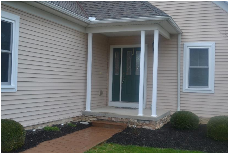
27. View of a typical stamped concrete entry walk and entry porch at a home.
