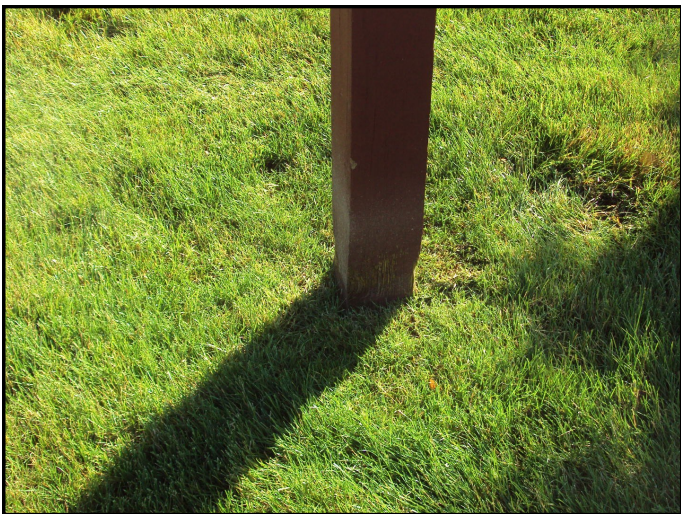
Trimmer Damage—Sign Post
