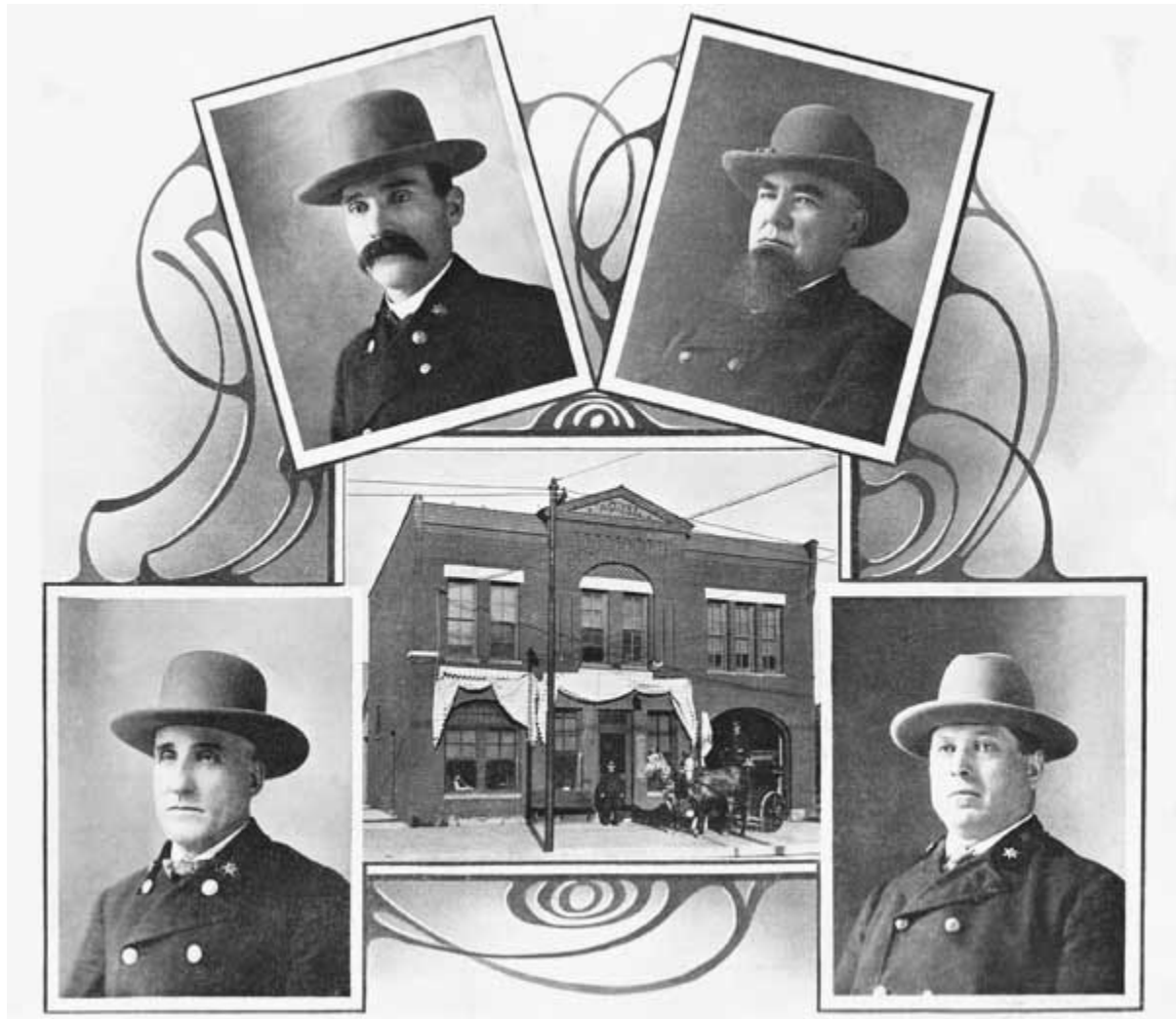
Ducas Street Substation and Officers
