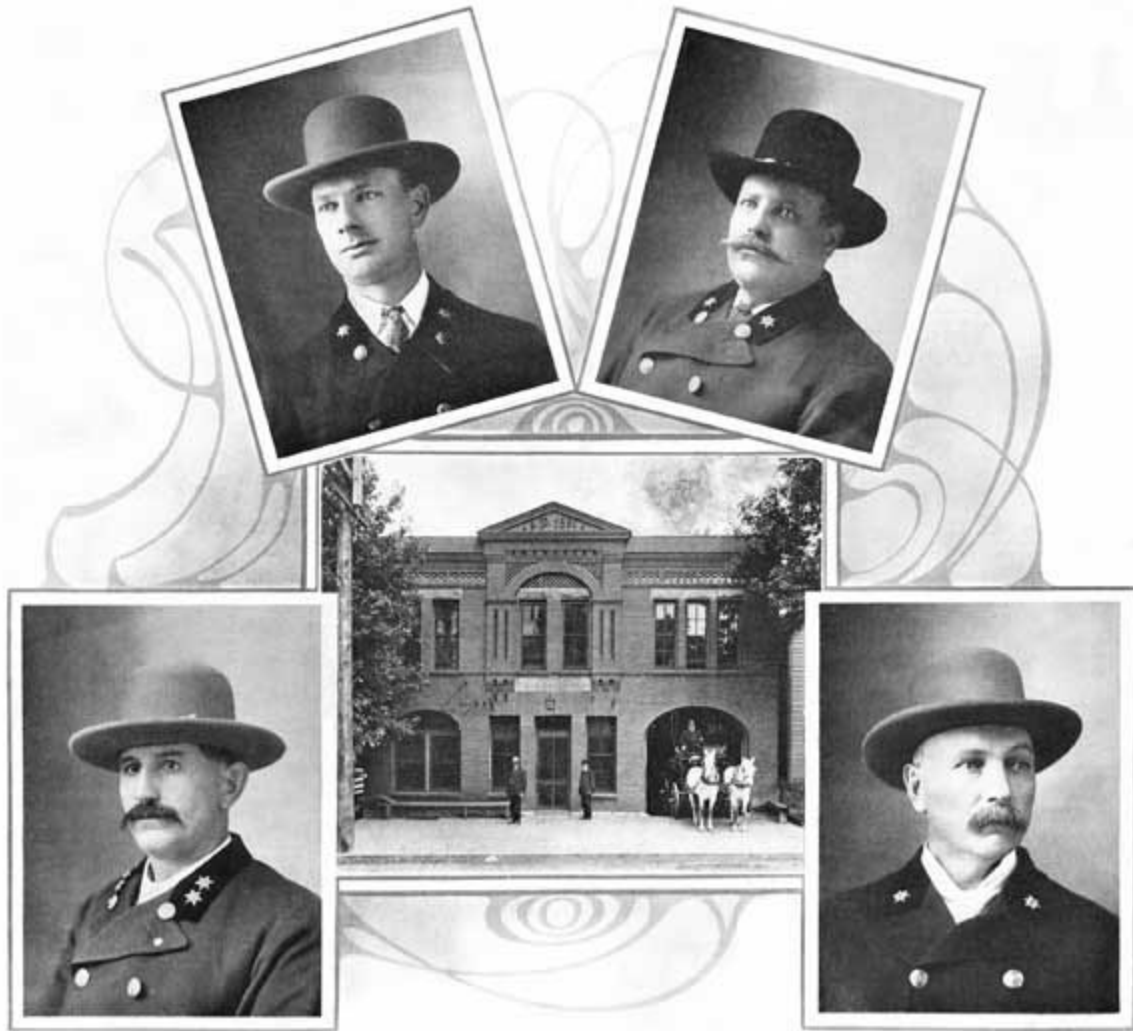
Margaret Street Substation and Officers
