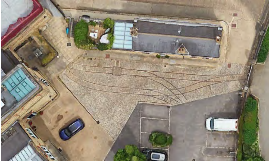
Figure 13 Satellite image showing the remaining of the original pavement and rails. The building on the top of the image is the Pump House Mater's Cottage (original building), now corresponding to nr. 7 Pump House Close.
