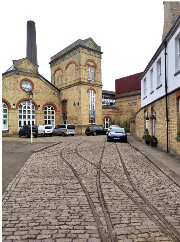
Figure 14 The communal courtyard as it appears today. The tall opening starting at ground floor level to the North-East façade of the Accumulator Tower was created with the conversion in 2001.
