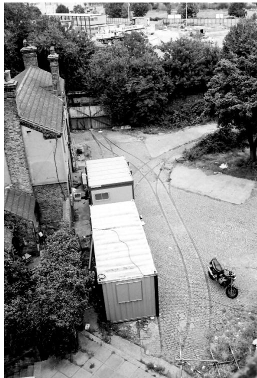
Figure 12 The yard to the south, before the conversion works (Tim R Smith, Greater London Industrial Archaeology Society, 1999), showing the Pump House Master's Cottage (currently 7 Pump House Close) to the left, and the 3-foot gauge tramway from Albion Dock, which entered the site through the gates at top left. The branch to the right led to the strategic coal store, which was added in 1907 to hold strategic reserve of coal in case of shortage of supply caused by, for example, strikes, and that has been demolished. Underneath the portacabin the tramway ran over a weighbridge. This photo has been probably taken from the water tank on the top of the Station Coal Store.
