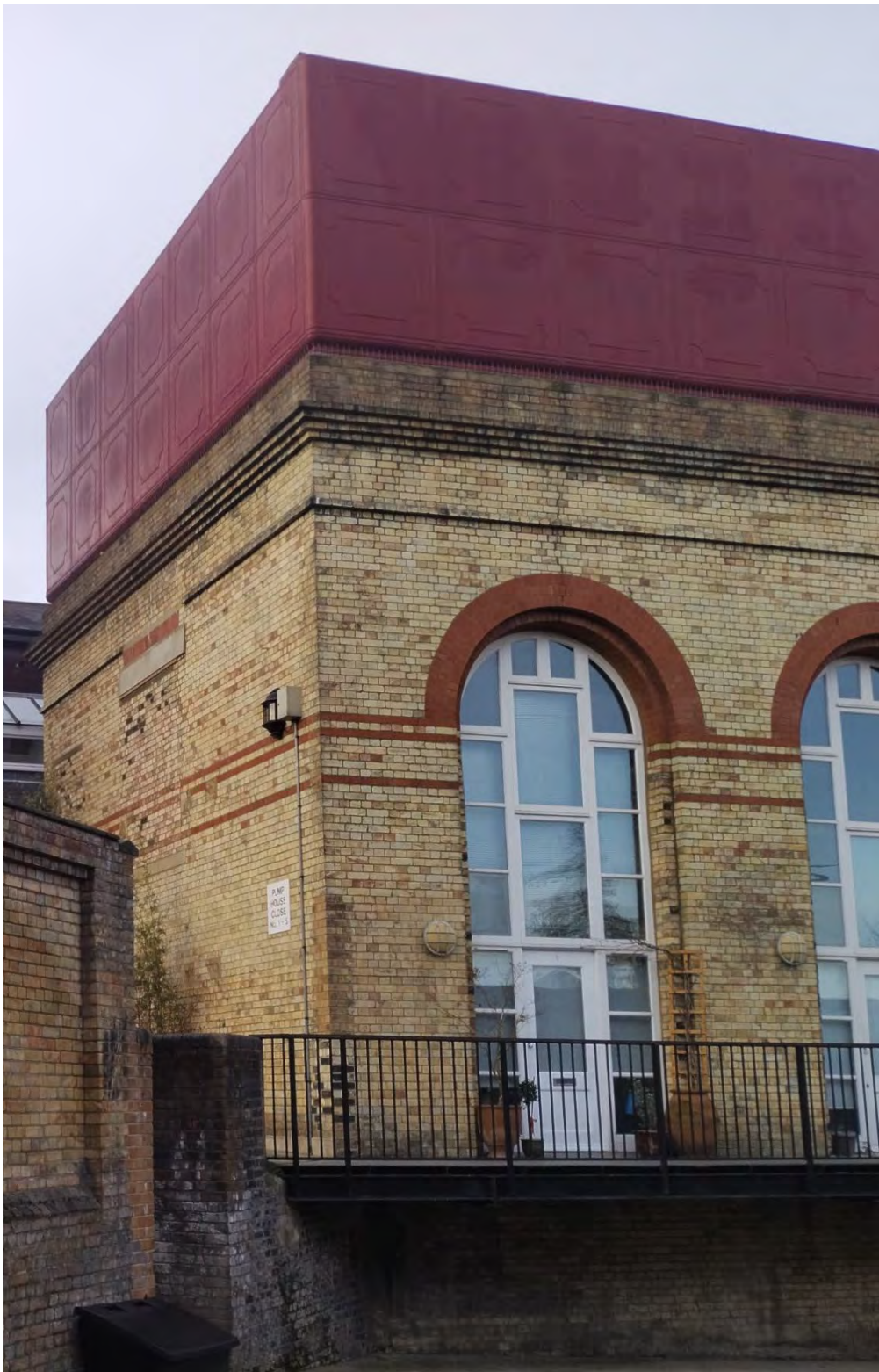
Figure 28: The original opening was with the sill at the level of the first course of red bricks, 9 courses below the start of the arch itself. The frame is not of significance as it is modern, and it has changed several times as shown by the photos taken in 1975 and 1999 and as illustrated in Figure 27.
