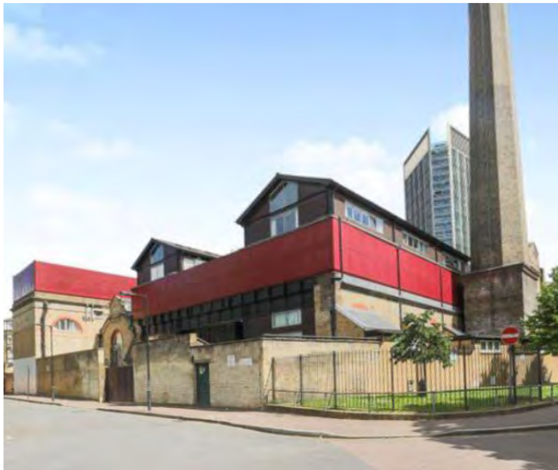
Figure 4: The two pitched-roof blocks added with the conversion viewed from Renforth street.
