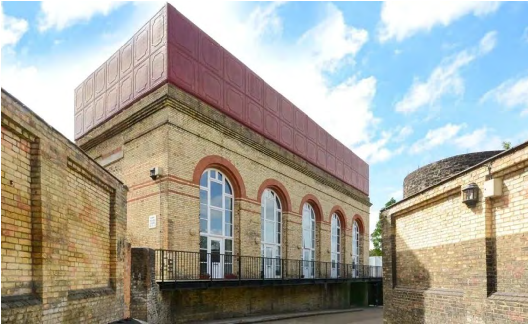
Figure 19 Besides the change of the opening's sill level (which has been dropped down to create the access), the design of the frame has been changed again, losing the curved and the radial elements at the top.
