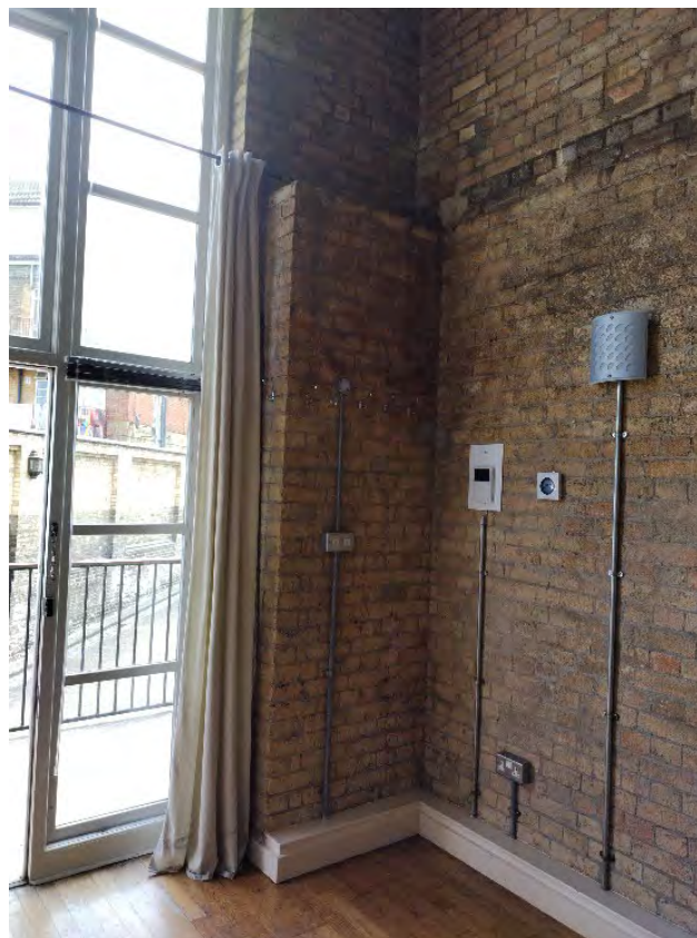
Figure 26: corner of the building with a brick pillar and marks on the wall which seems suggesting the presence of a mezzanine level.
