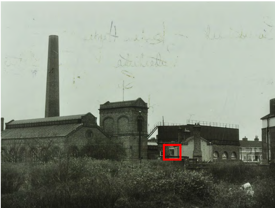
Figure 20 Rotherhithe Pumping Station, Swan Road: exterior, 1975, © London Metropolitan Archives (City of London). In the red square, the opening to the side façade of the Coal Store, which at the time had glazed frames. To be noted: the opening seems to be square rather than rectangular and the concrete lintel is already in place.
