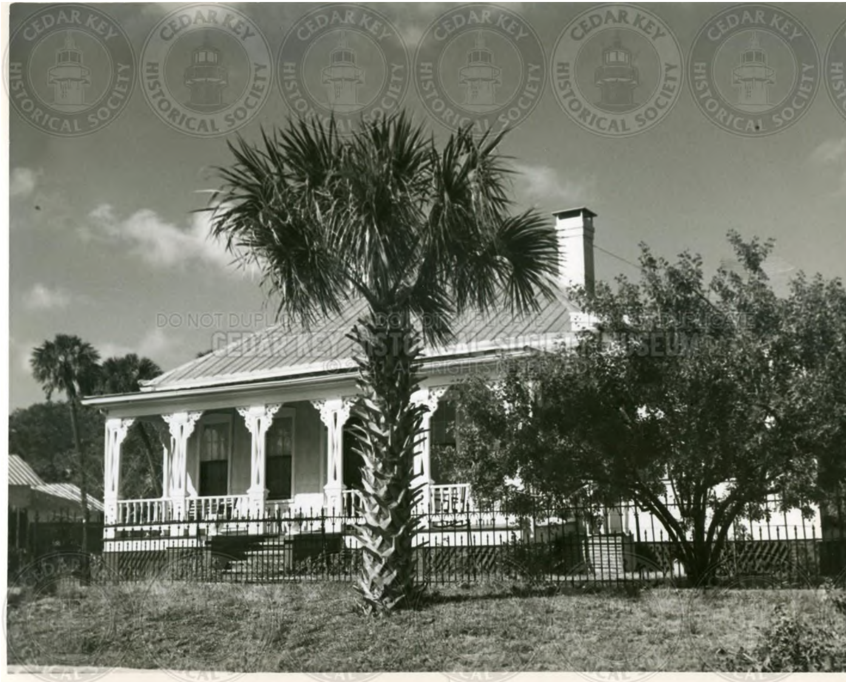
IMG11043 BOAZ C. WADLEY HOUSE
