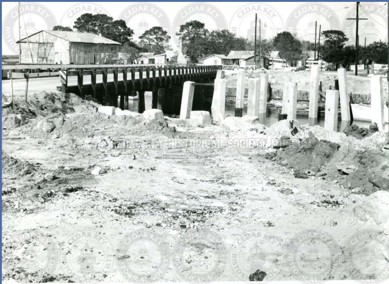
IMG03002 BRIDGE, LOOKING NORTH, STATE RD. 24
