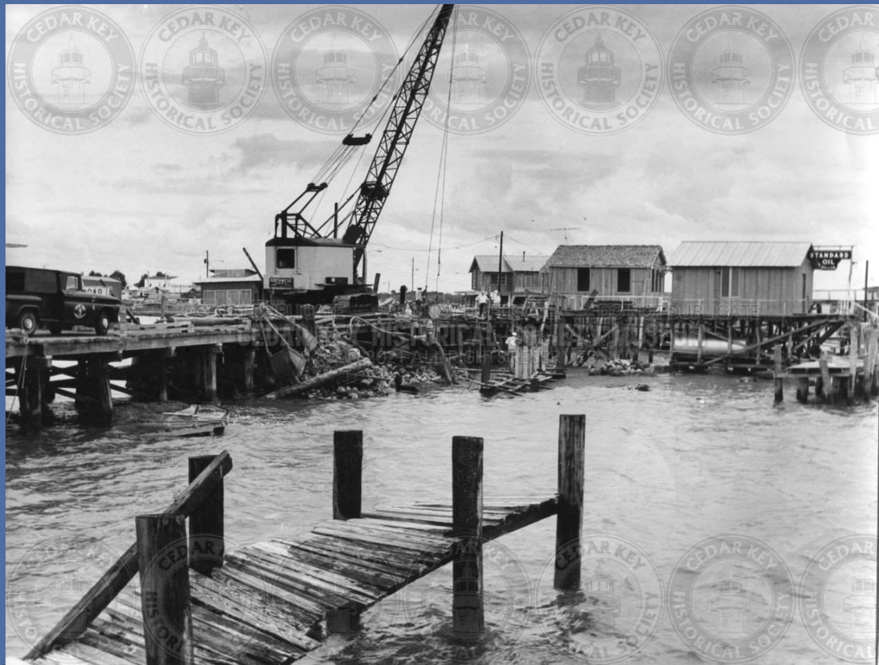
IMG03016 DOCK CONSTRUCTION, LOOKING WEST
