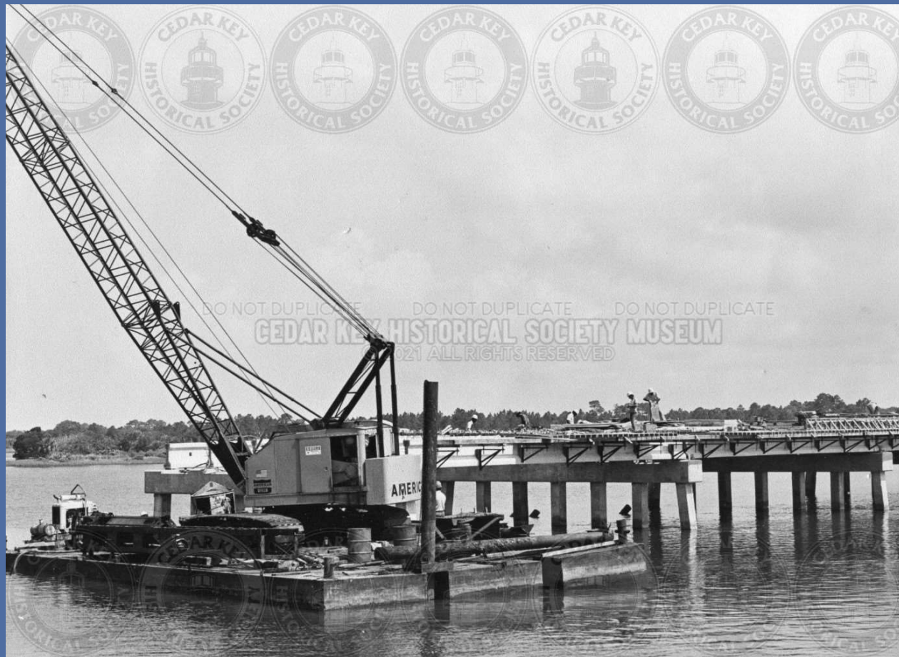
IMG03010 CONSTRUCTION OF NEW NO. 4 BRIDGE, 1974
