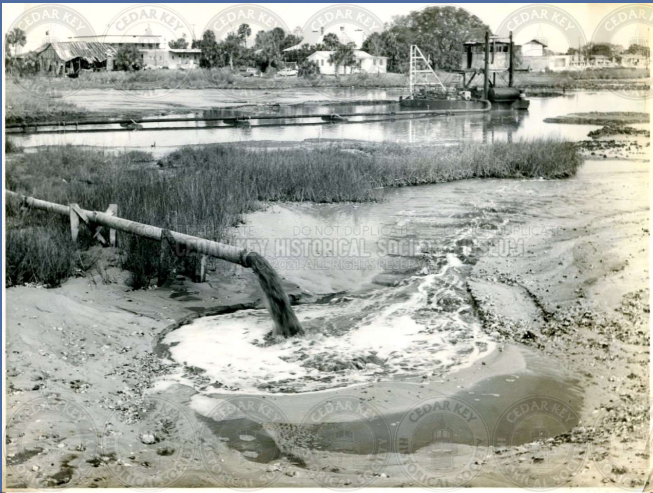
IMG03042 BIG DOCK LOOKING EAST, 1949
