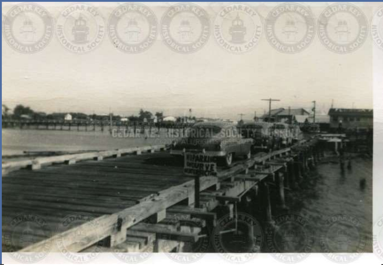
IMG03047 CA. 1932-35, BUILDING OF BIG DOCK
