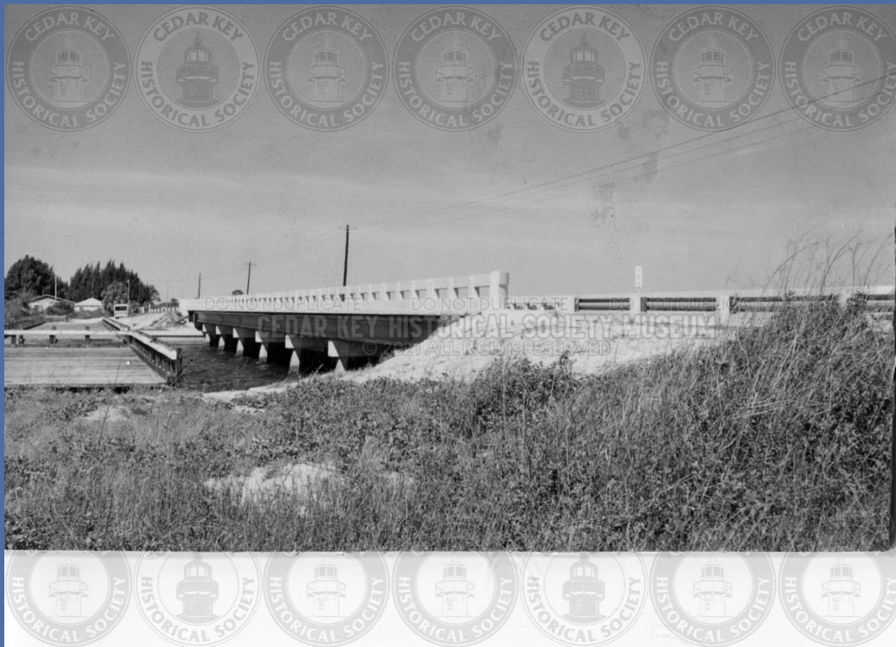
IMG03009 NO. 3 BRIDGE
