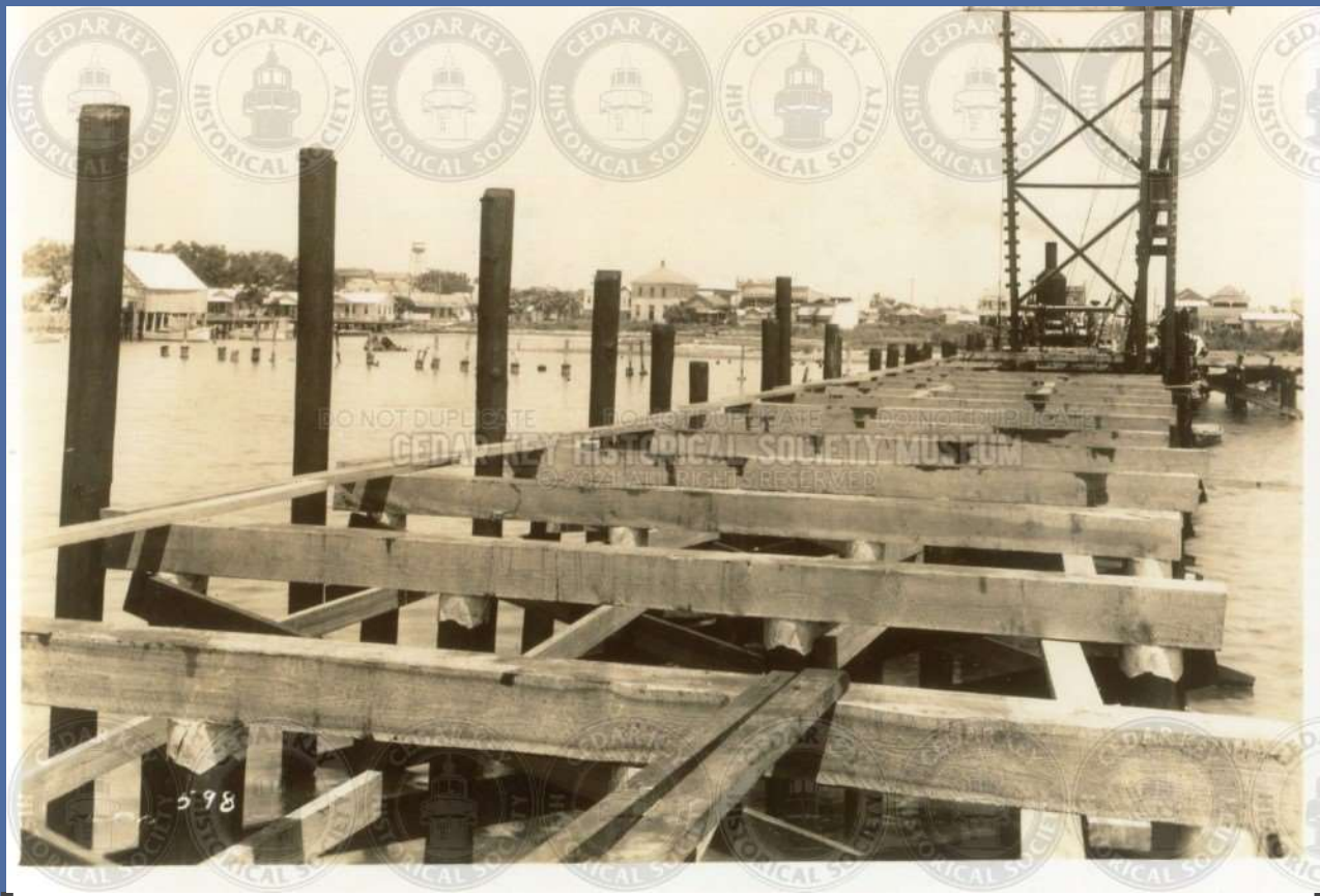
IMG03028 BIG DOCK UNDER CONSTRUCTION
