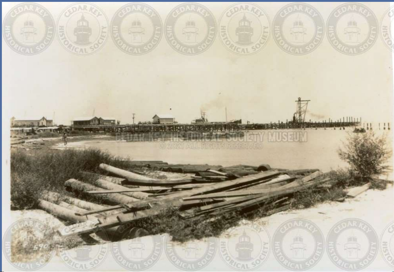
IMG03041 RED BRIDGE, HWY. 24 & 3RD ST., EARLY 1900S
