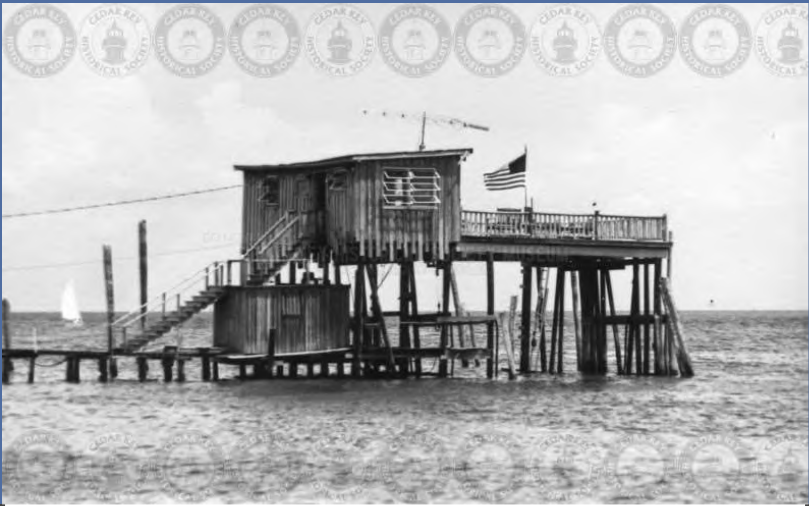
IMG18075 IMG01116 THOMAS'S GUEST HOUSE
