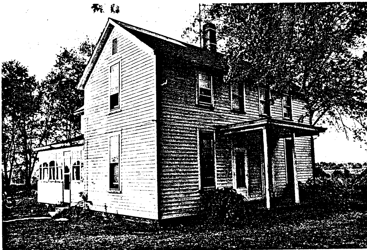
Figure 15.—Test structure 19, near a coal mine.
