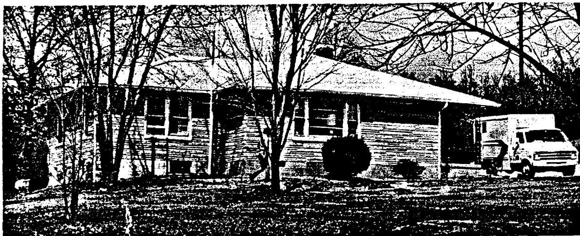
Figure 24.—Test structure 30, near a coal mine.
