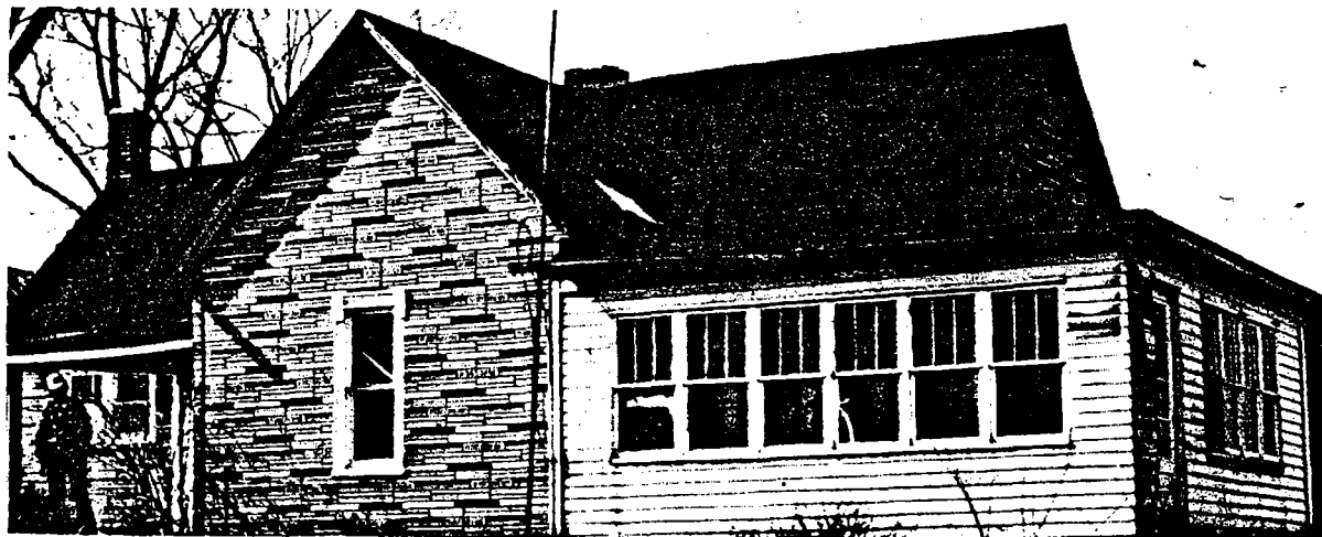
Figure 21.—Test structure 27, near a coal mine.
