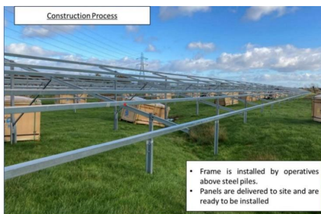
Figure 9 Photograph showing the framework system prior to bolting on the panels.
