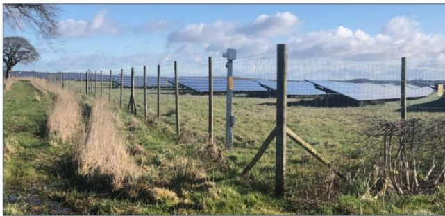
Figure 10 Photograph showing the typical specification of a stock proof security fence and security cameras
