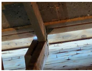
Roof to wall connection
