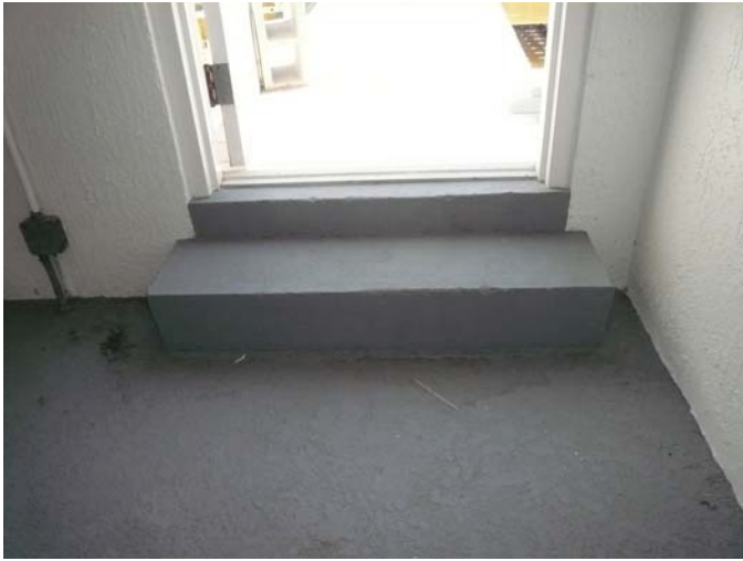
Concrete roof deck
