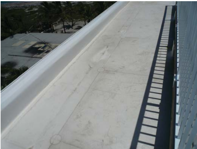
Membrane roofing
