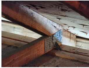
Roof to wall connection
