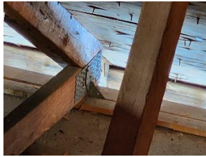
Roof to wall connection
