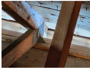
Roof to wall connection
