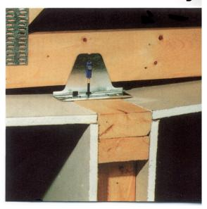
**With Truss Floater Bracket**
