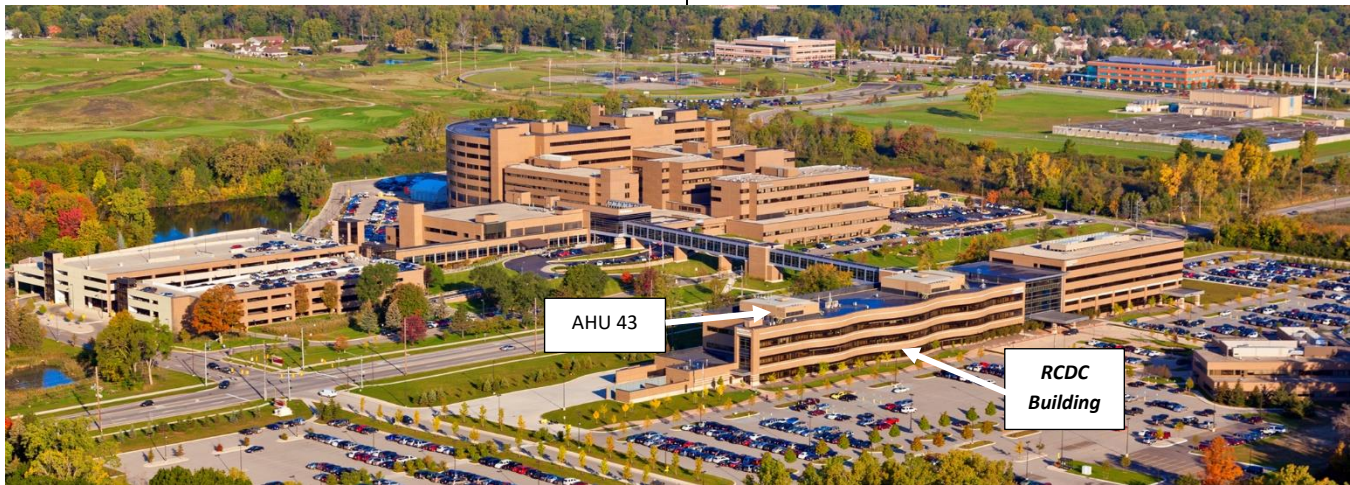
Aerial View of Major North Central US Health Systems Facility, Showing RC/DC Building and AHU-43 on the Roof
