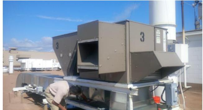
*GUE Electrician makes airflow temperature measurements on the 12.5 Ton York Unit*
