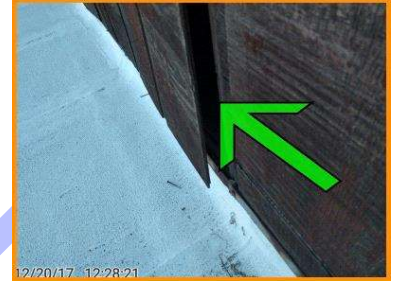
12/20/17 12:28:21 Garage, at the roof - Roof Wall Connection
