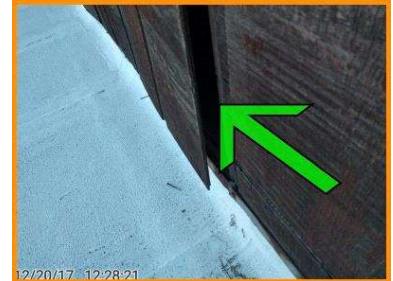
12/20/17 12:28:21 Garage, at the roof - Roof Wall Connection
